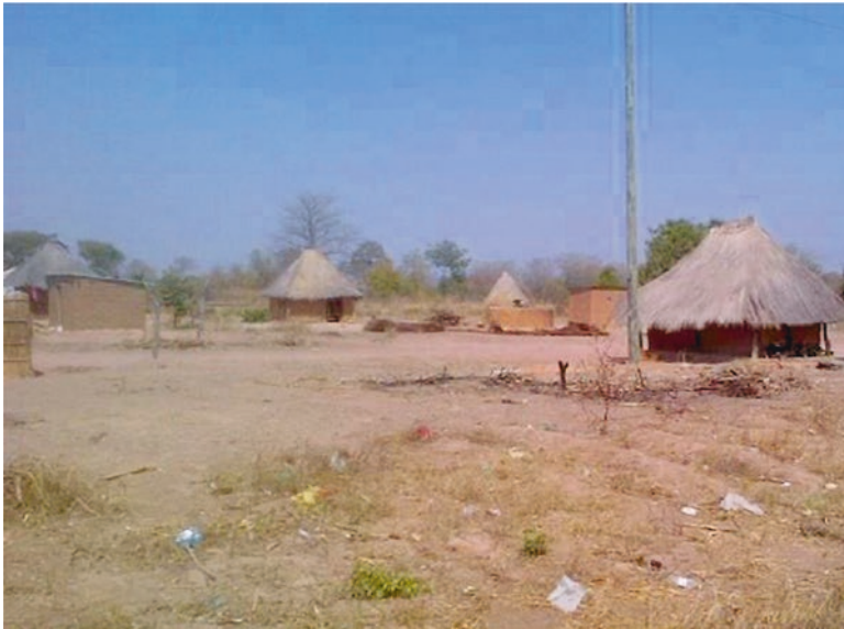
Fig. 17.2 Typical rural housing in Africa and many other developing countries, consisting of mud brick walls with roofs of generations-old, tinder-dry thatch or sheet metal held down by stones. The walls do not contain wiring or plumbing, and these buildings are not considered lightning safe. (2015 Zambia photo ©M.A. Cooper)
